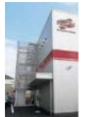
[Outdoor upstairs to rooftop] 49
